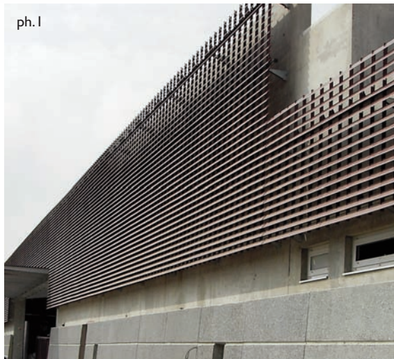
Station épuration - Lattes (34)
